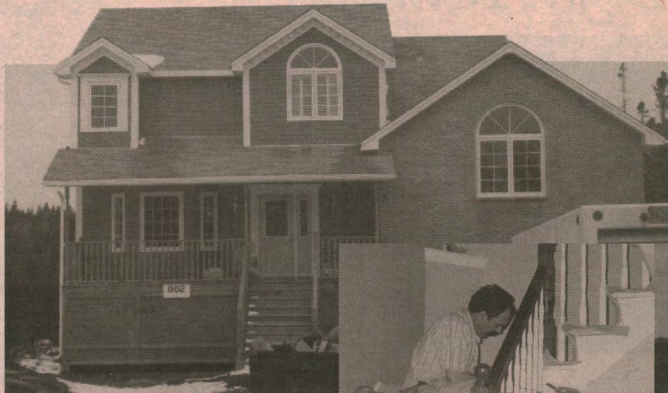
Above: Just before the grand opening: University House 96, located at 862 Kingswood Drive, Kingswood On The Lakes Subdivision.
