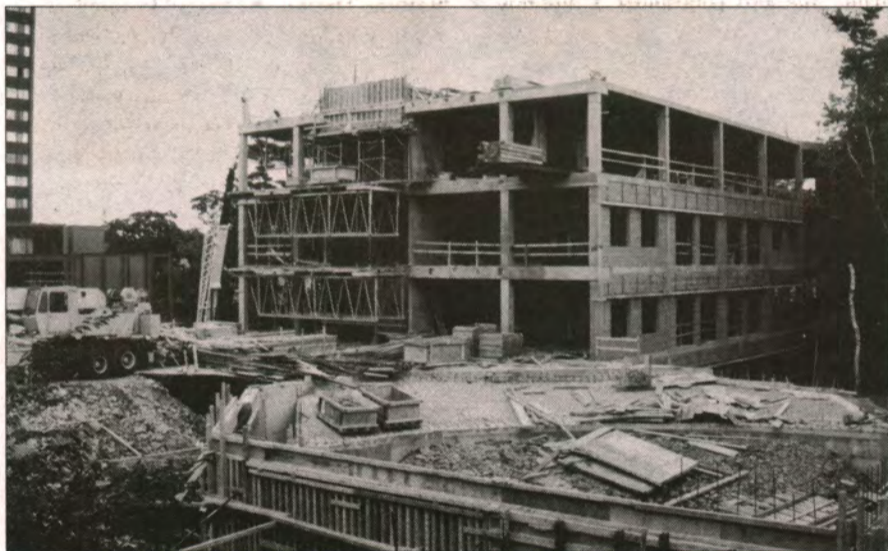
The construction process for the building is moving quickly.
