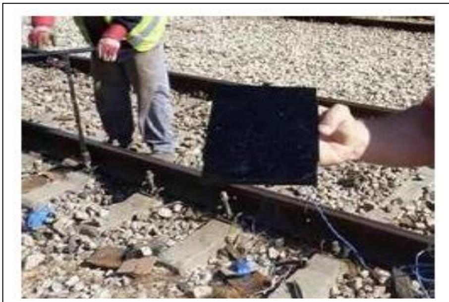
Figure 7. - Installing piezoelectric pads by Innowattech Inc. on Israeli railways.
